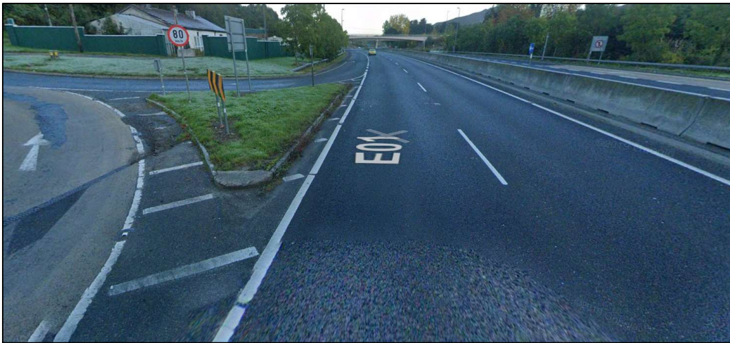
Figure 5 Abrupt removal of hard shoulder – N11 northbound at Junction 9 (Glenview) (© 2021 Google)
