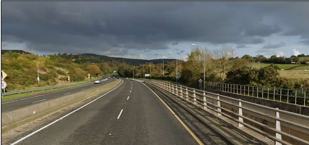
Figure 4 Narrowed hard shoulder – N11 southbound at Junction 11 (Kilpedder) (© 2021 Google)
