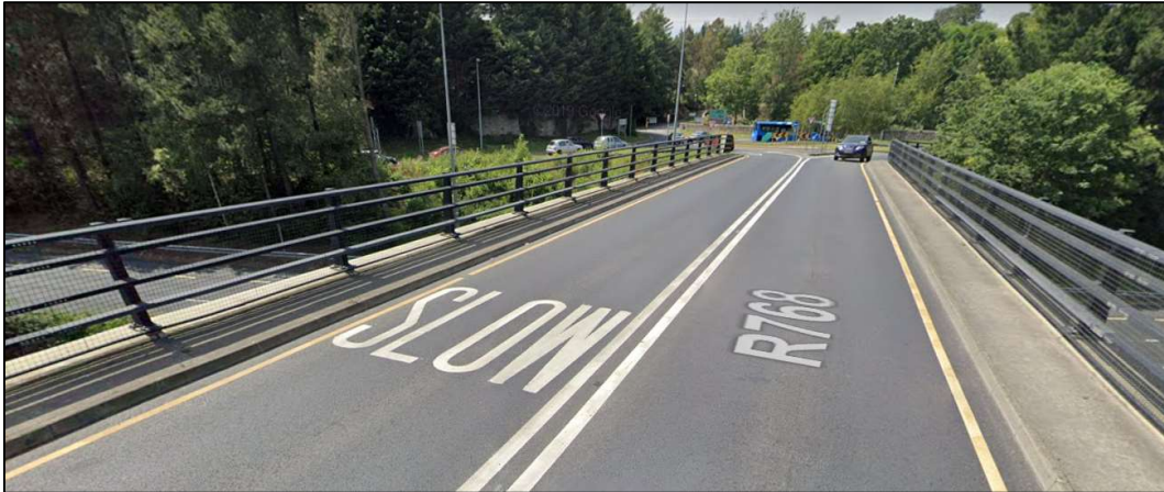
Figure 6 Absence of pedestrian/cyclist facilities – existing R768 overbridge at Junction 7 (Bray South) (© 2021 Google)
